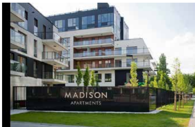
Madison Apartments - Poland - Clima Canal
